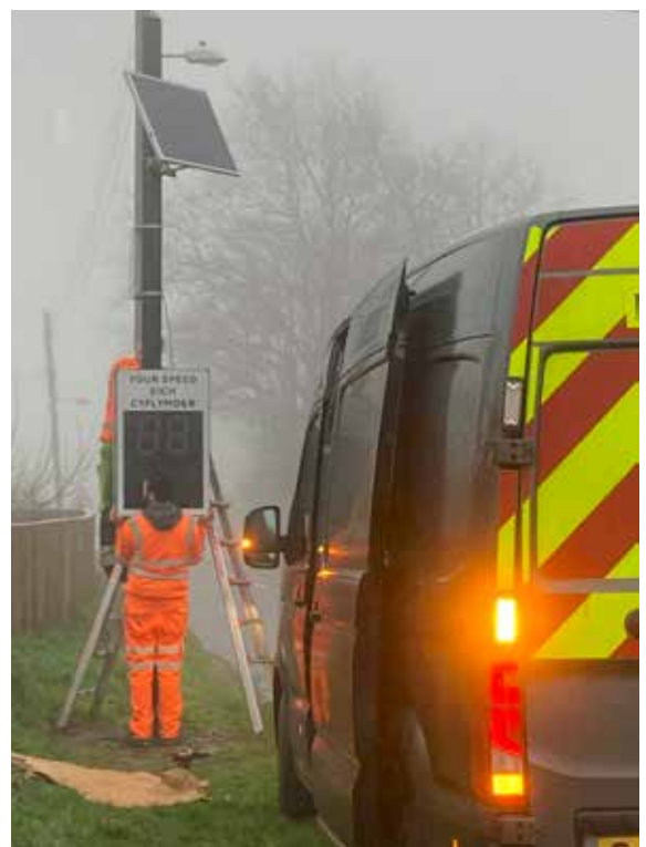
Installation: the weather was not too good!
